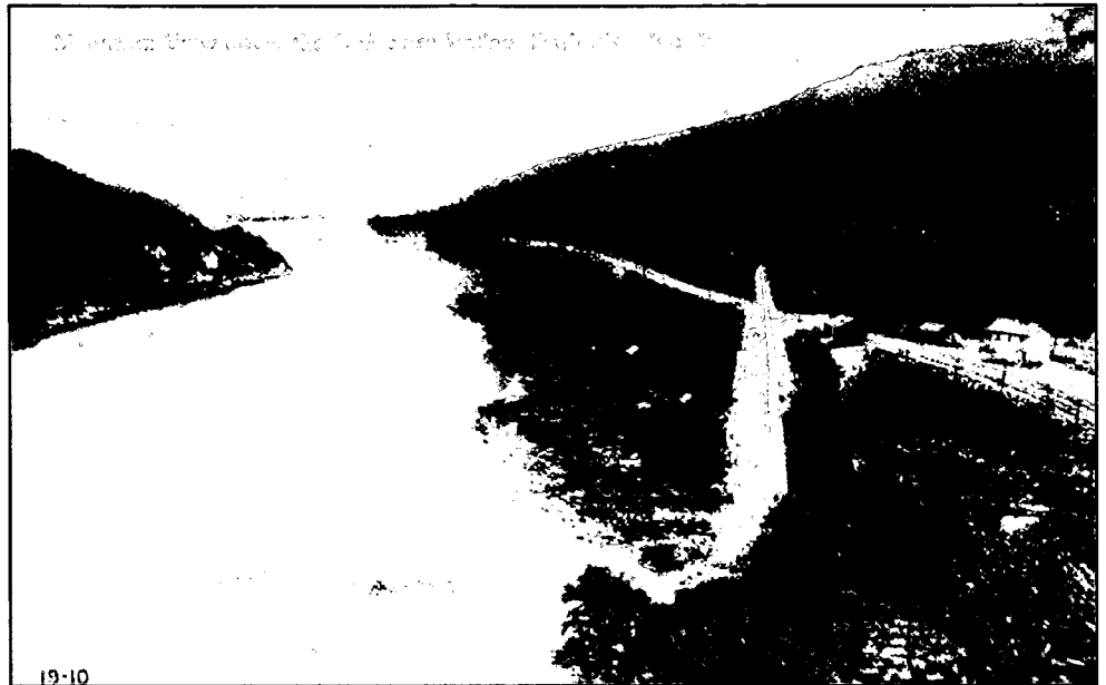
The Erie Railroad ran Walker Lake Falls, an 80-foot waterfall, into a pipe in order to deliver water to the railroad in Parker's Glen, Pennsylvania. The hydraulic head from the fall of the water created this spectacular fountain. John F. Kilgour, the "Bluestone King," founded Parker's Glen in 1875 as a mining community for the Parker-Kilgour Stone Mills. Bluestone, a type of flagstone, was quarried in the upper Delaware for sidewalks and curbing. Today, Parker's Glen is one of several towns on the upper Delaware River that has disappeared. (Excerpted from Along the Delaware River )
