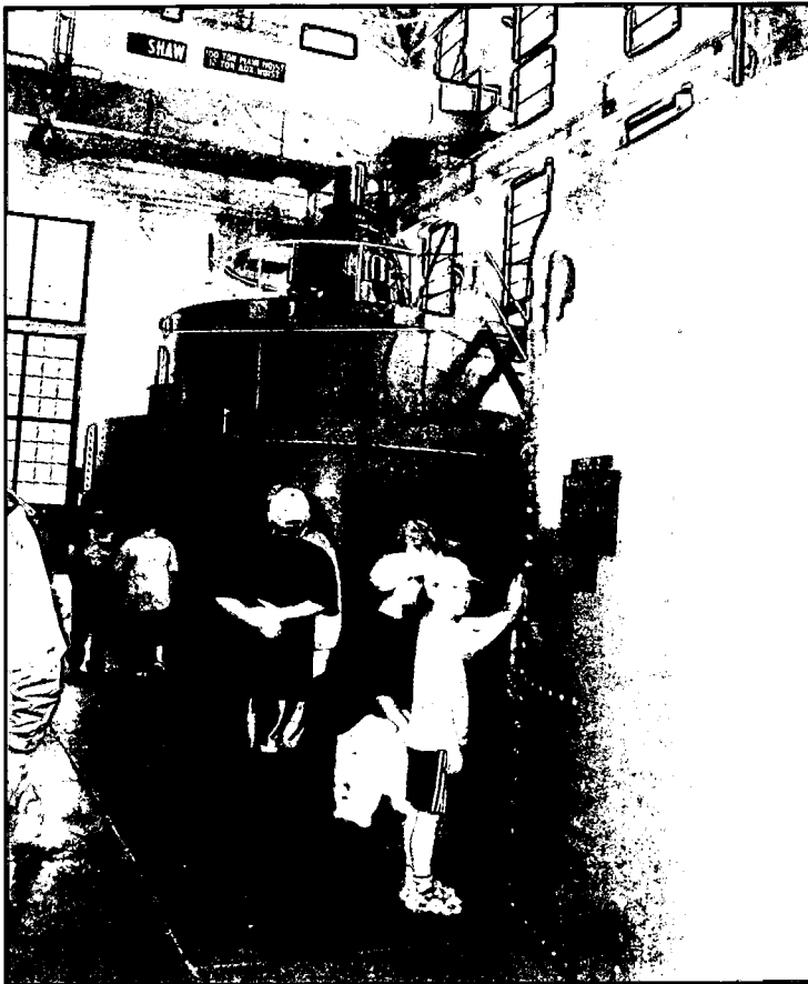
FEEL THE POWER: Boys on the August 25 open house tour of PPL Generation's three-story power house in Hawley, PA feel the vibrations from a Westinghouse generator as water piped 3.5 miles downhill from Lake Wallenpaupack rotates underground turbines, which then spin the generators to produce up to 44,000 kilowatts of electricity, enough to power about 35,000 homes. (UDC Photo by Laurie Ramie)
