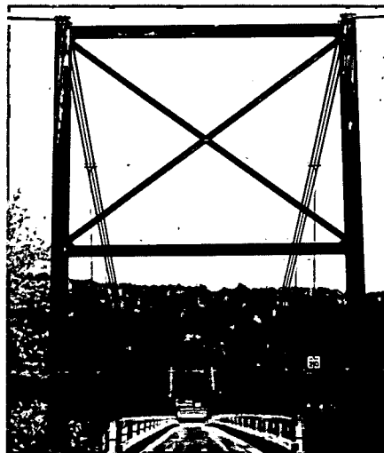
The Kellams-Stalker Bridge. Photo by Dave Soete.
