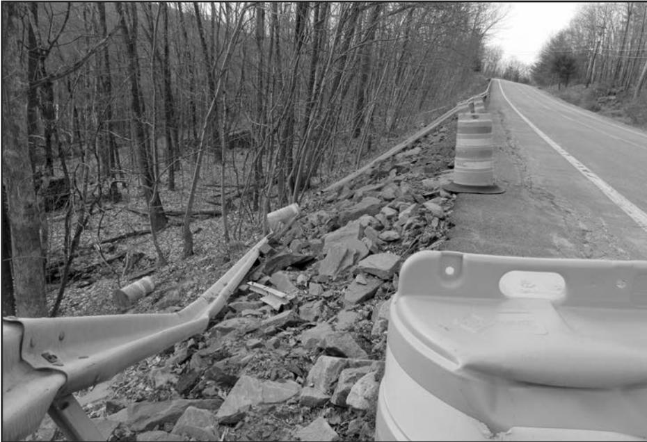
**MOTOR SAFETY:** This guide rail section on New York State Route 97 in the Town of Delaware has failed, with many of the orange barrels placed there by the Department of Transportation as a safety precaution also rolling down the steep slope. (UDC Photo by Laurie Ramie)
